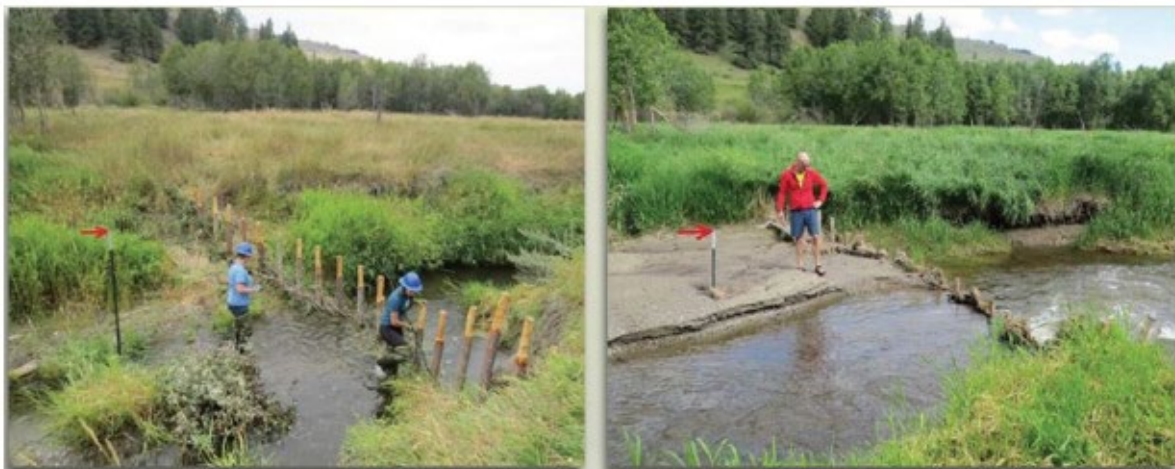
Figure 10. Sediment retention by a BDA on Triple Creek. Note the arrow pointing to the top of the same staff gage in both photos. Photo credit: Okanogan Highlands Alliance.
